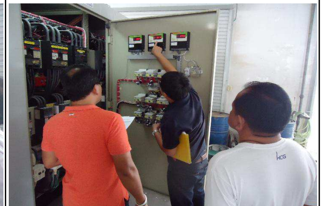
IEMS System installation inspection and acceptance
