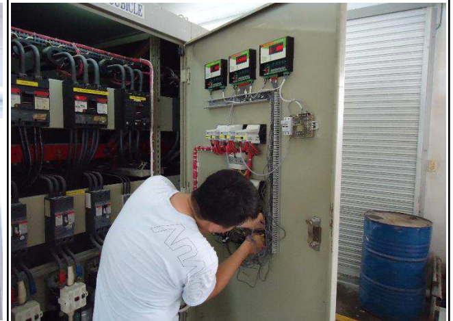
Split CT installation
