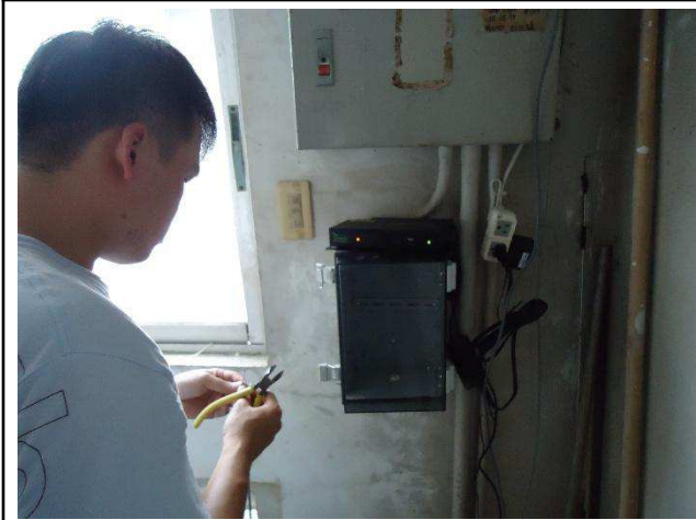
Smart Gateway installation
