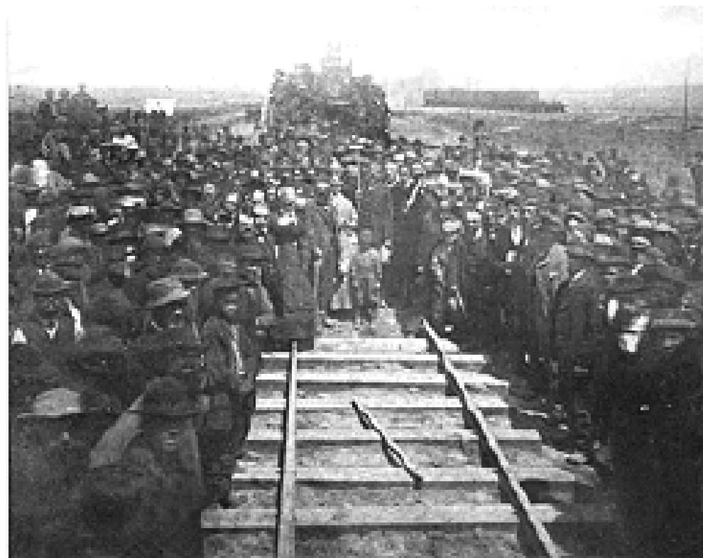
The Last Rail is Laid
